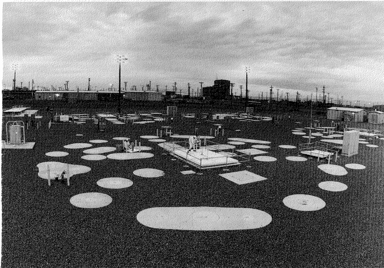
HIGH-LEVEL NUCLEAR WASTE TANK sits about three meters underground. Ports and risers admit instruments for monitoring and sampling of the waste. These entry tubes are normally sealed by the plates visible in the photograph.
