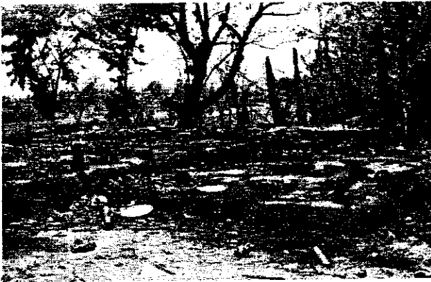
Burned house in the village of Pujgang.
